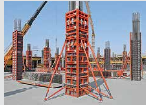
Column Formwork
