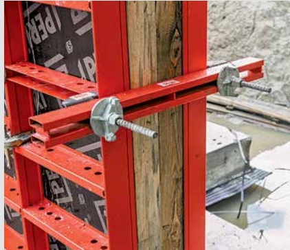
The simple stopend formwork with timber and filler plates.
