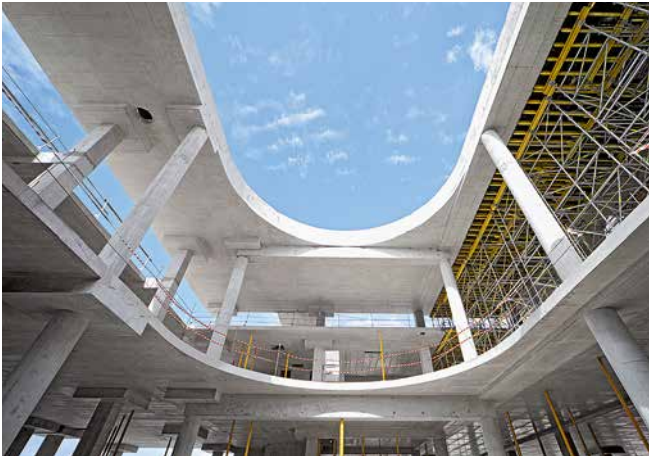
The 30 cm thick reinforced concrete slab was formed with MULTIFLEX.
