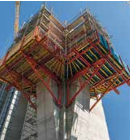
Horizontally mounted Brace Frame system combined with system components of the VARIOKIT Engineering Construction Kit form cantilevered working platforms.
