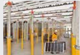
Slab Formwork
