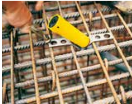
With the V-Tie Holder, as a lost part, an exact alignment of the Tension Anchor to 45 ° is possible.
