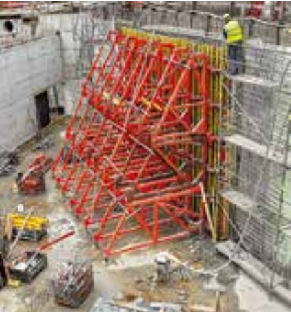
Force is safely and reliably transferred at all connection points of the SB-A0, A, B and C.
